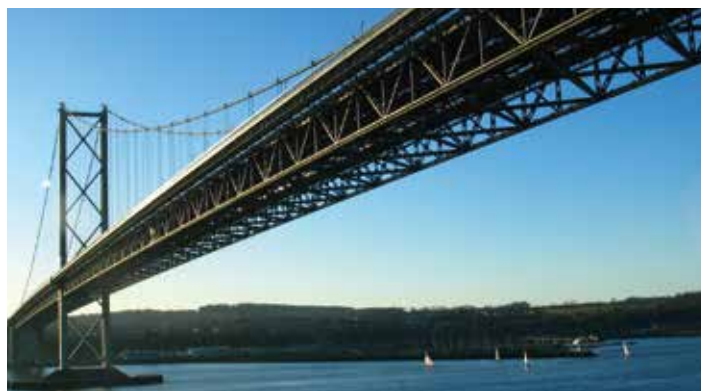
Forth Road Bridge
